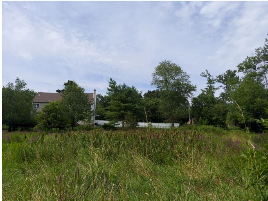
Photo No. 5: Basin Overall
