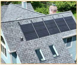
vastly improved their efficiency levels, and because shingles can be installed without roof penetration, solar shingles are gaining in popularity.
