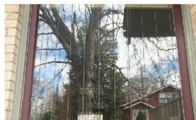
You can make a Zen wind curtain with cord, or anything that will hang in front of the glass at 4" intervals. Photo by Lisa Welch
